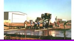
Trenching, plumbing, anchor bolts placed and concrete poured 9/2008
