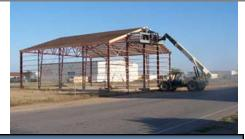
Frame attached to anchor bolts and trusses for roof installed 3/2009
